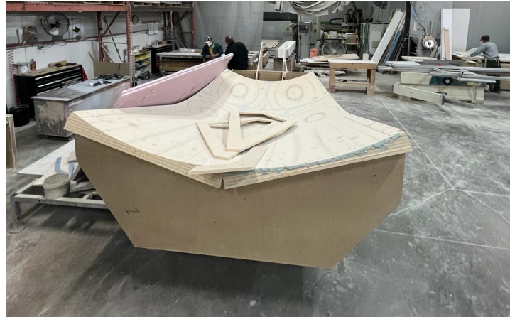
Image: Wooden mold for Mosque Dome
