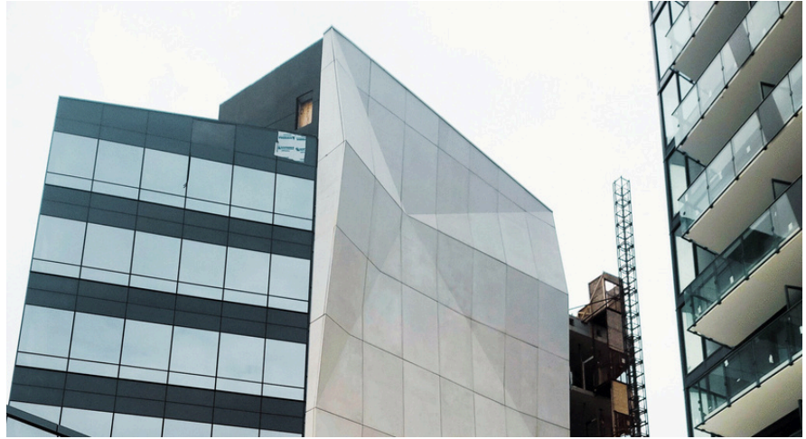
Dynamic Building Envelope | Ellie Tower Condominium Toronto | Canada
